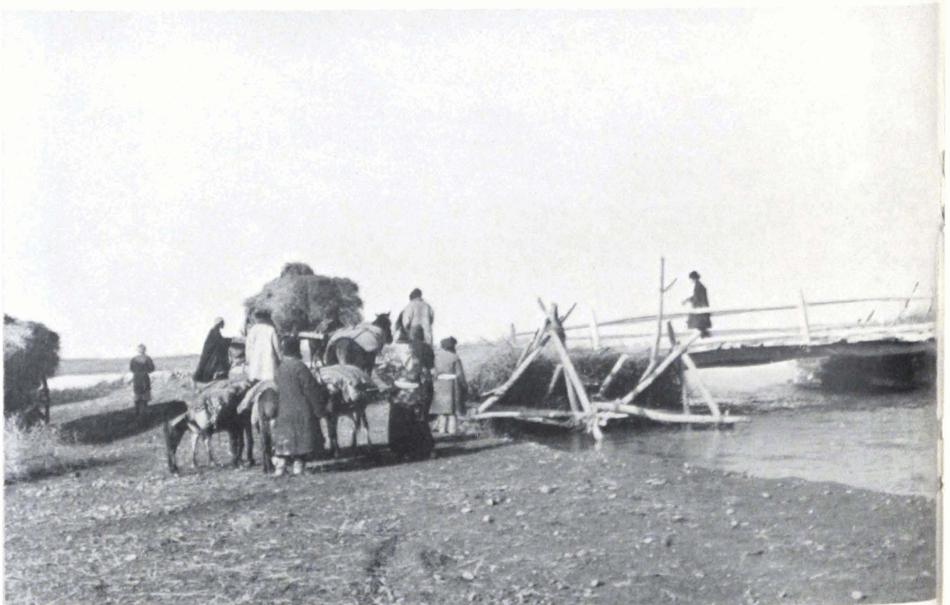
Bridge Over the Aksu River
