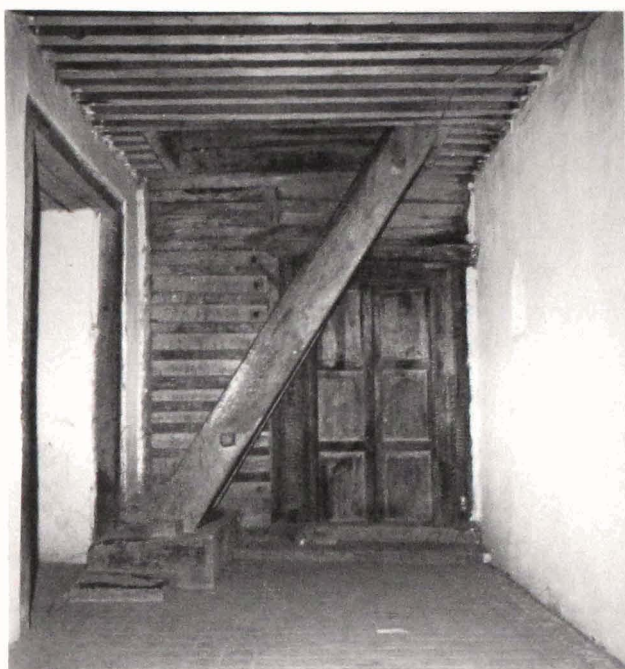
53. Room S1-2, first floor
