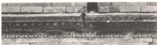
Fig. 1-1-10. Cornice above the second floor, the Gharat
