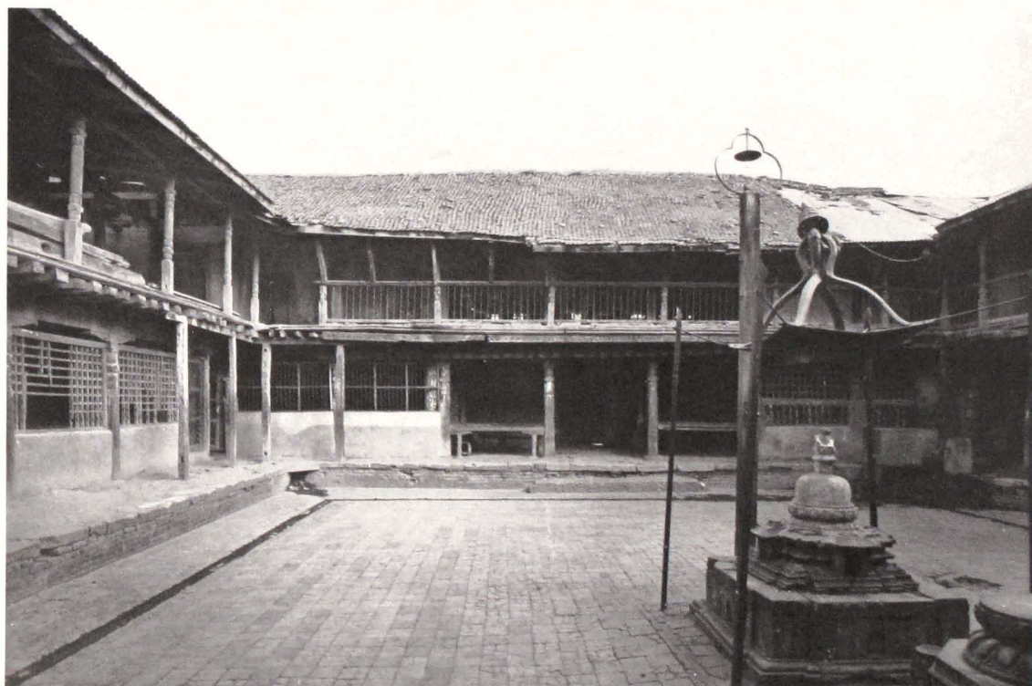
74. Courtyard and east wing
