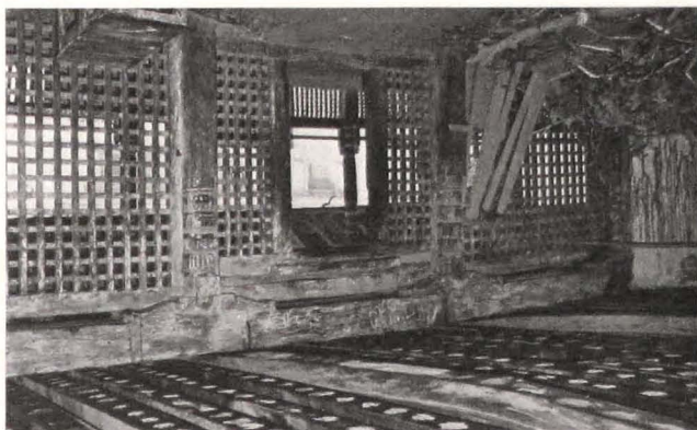
92. Courtyard and east wing
