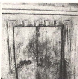
Fig. 2-3-14. Doorway, second floor, Charumati Vihara
