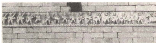
Fig. 1-1-11. Cornice within the second floor, the Gharat
