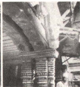
Fig. 2-3-12. Circular pillar, Dalan, north wing, Sundari Chok, Patan Darbar
