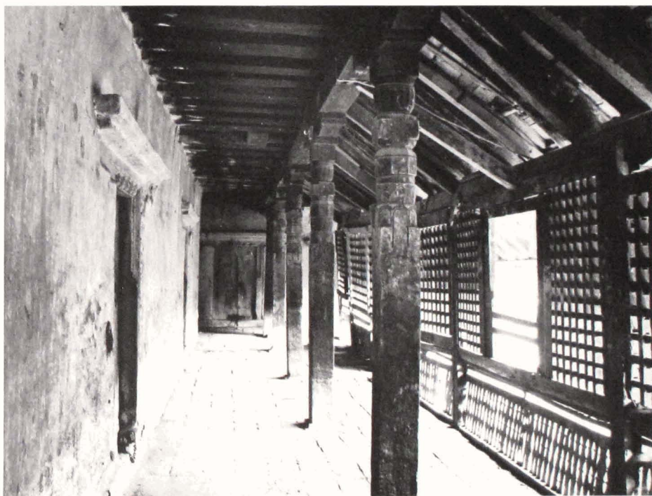
90. Second floor, east wing
