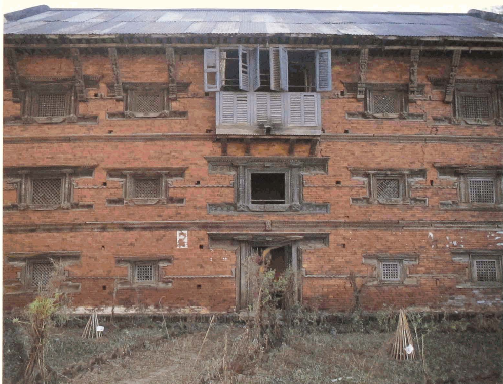
8. West façade, Ranga Mahal
