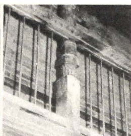
Fig. 1-3-29. Lower part of pillar, balcony, I Baha Bahi
