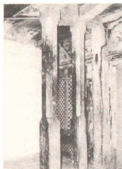
Fig. 1-1-19. East window (3W-2) of room S3-1
