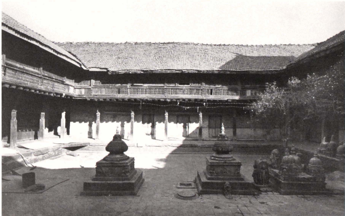
85. Courtyard and east wing
