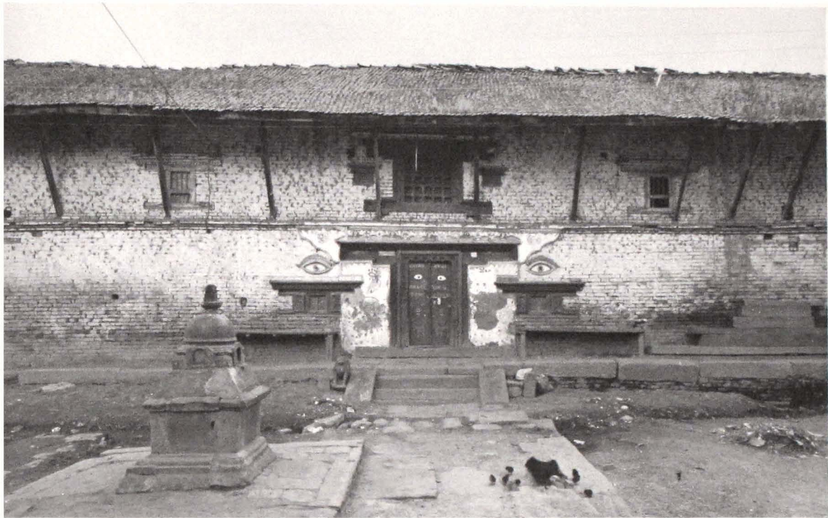
84. Front entrance, north façade
