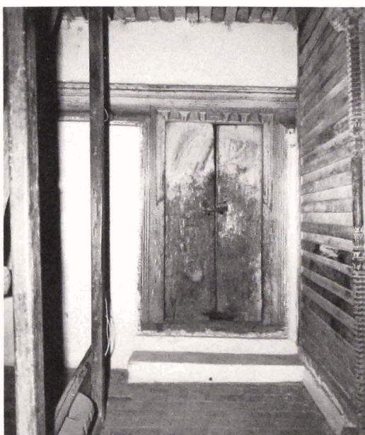
54. Room S2-3, second floor
