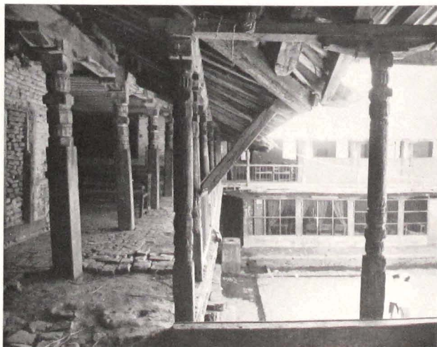
83. Balcony, second floor
