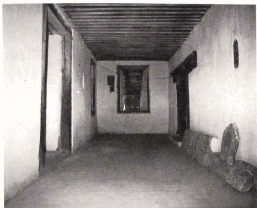
52. Room S1-1, first floor
