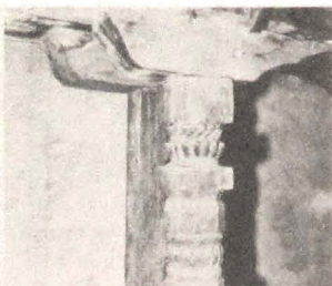
Fig. 2-3-8. Ancient pillar (recycled), Mul Chok, Patan Darbar
