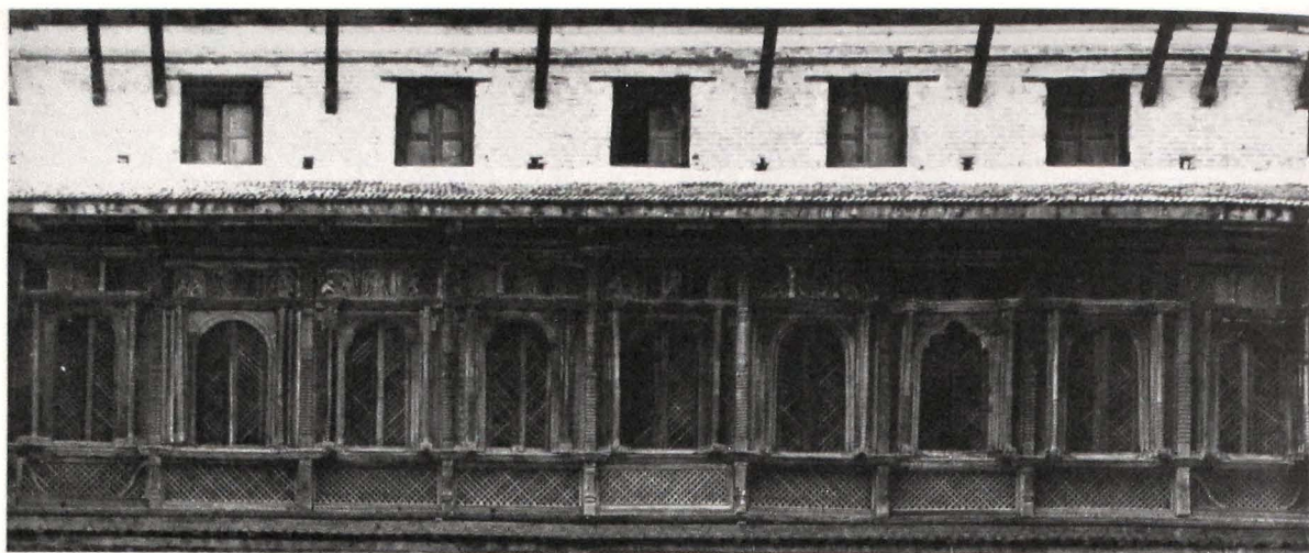
48. Windows, fourth and fifth floors, east façade
