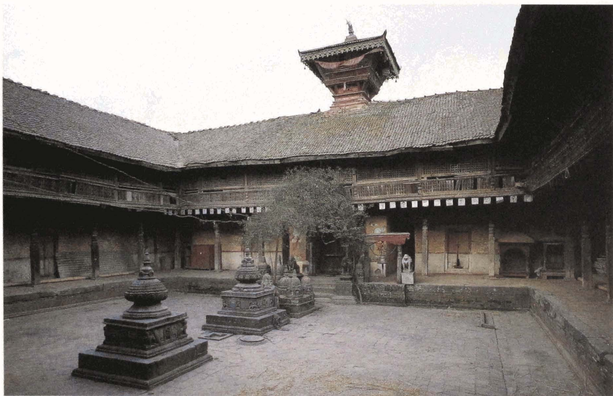
20. Courtyard and south wing, Charumati Vihara, Deo Patan
