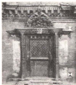
Fig. 2-3-11. Circular pillars supporting the Torana, entrance of the Mul Chok , Patan Darbar
