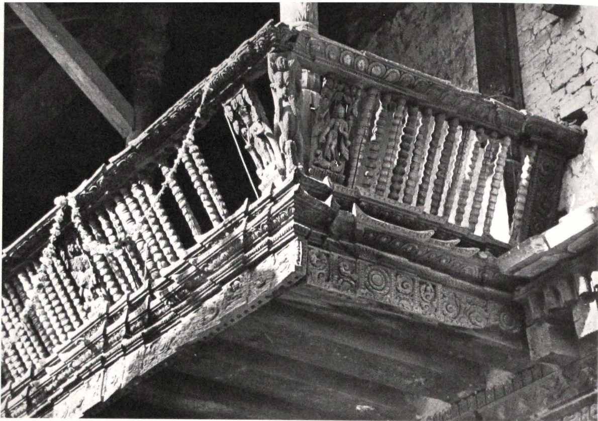
81. Balcony detail, east façade
