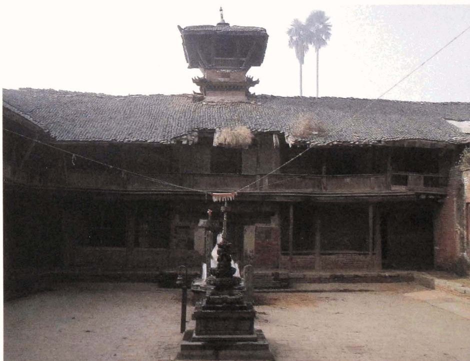
22. Courtyard and south wing, Jya Baha Bahi, Patan
