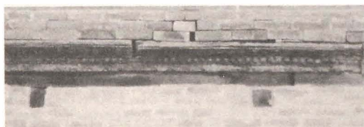
Fig. 1-1-7. Cornice above the first floor, Sattale Darbar
