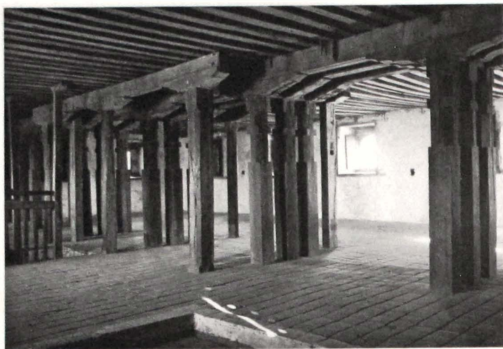
57. Room S5-1, fifth floor
