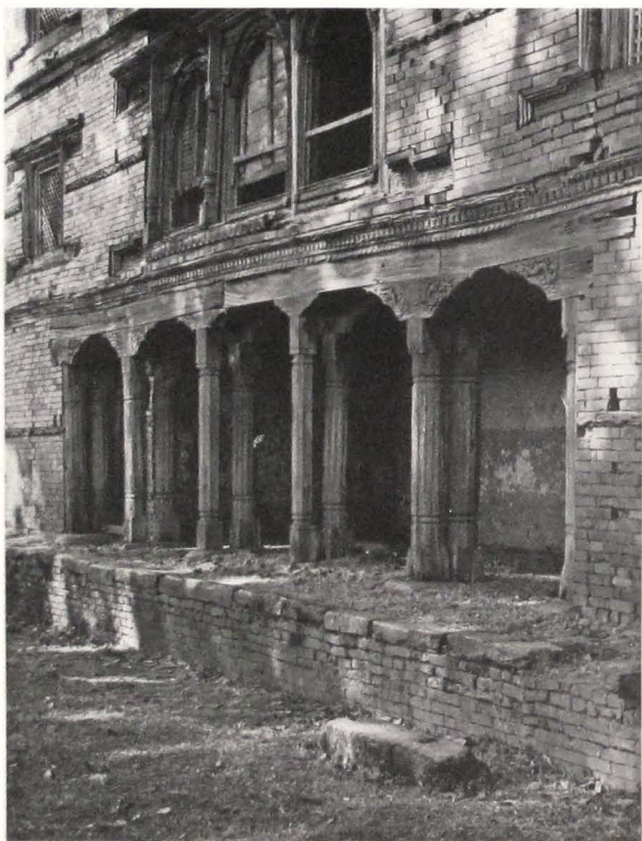
65. Dalan, east façade
