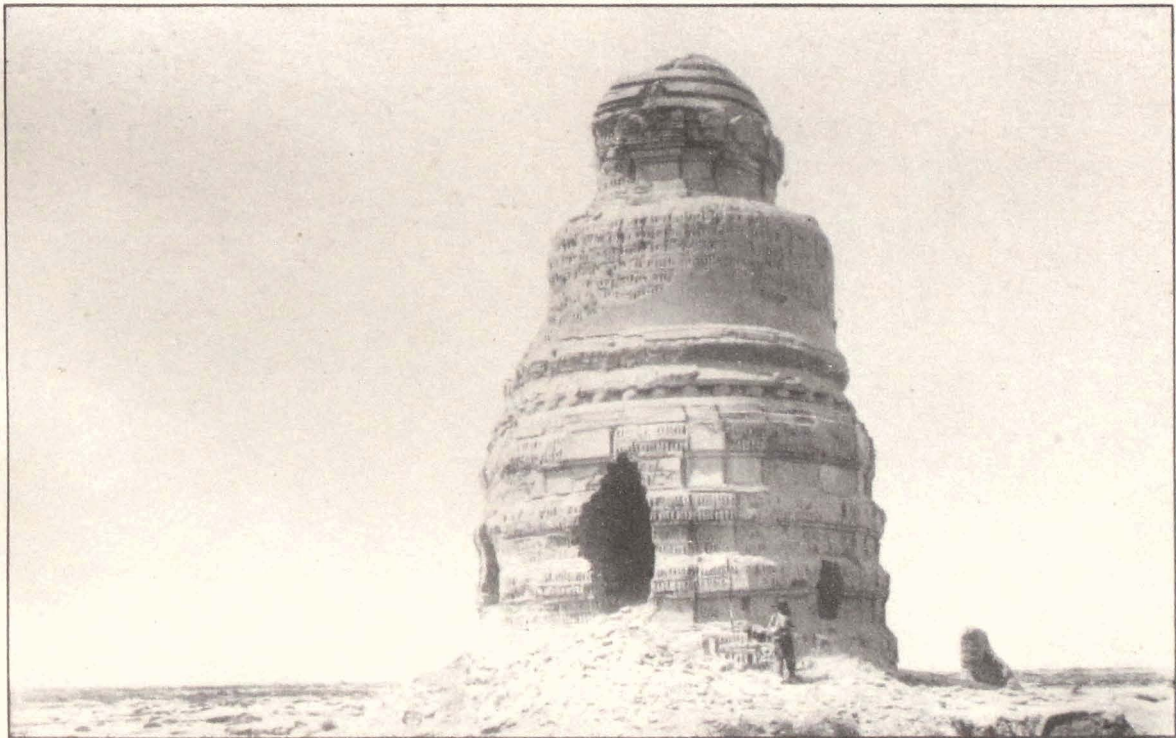
238. RUIN OF MAIN STŪPA, EAST OF SO-YANG-CH'ENG, SEEN FROM SOUTH.
