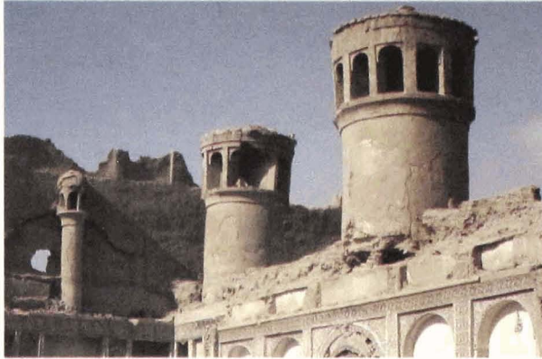
Omnidirectional bad-gir in the ruins of a large, stately house in Herat.
