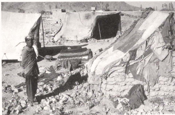
8. Encampment of Jat cotton tents on the edge of Kabul. Tent at left erected on initial settlement, while tent at right demonstrates the gradual transformation of the structure into a simple mud house by adding ever higher walls.
