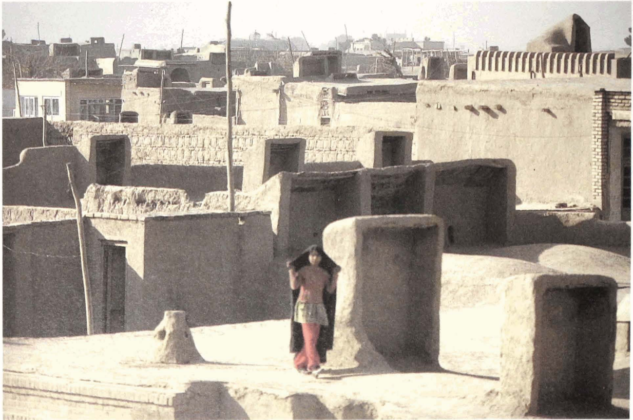
Rectangular bad-gir used in Herat on flat-roofed buildings.
