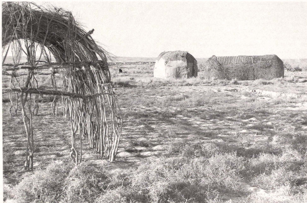
24. The three stages of construction of an ovate-oblong kadik hut in Sehyak, southwestern Afghanistan: at left, tamarisk framework; at right, mat covering applied to frame; in center, mud plaster applied to mat work.
