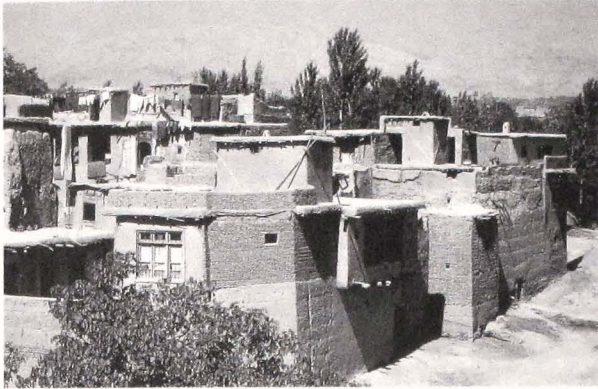
39. A village of multistoried houses south of Charikar employing composite construction including senj , a technique which uses a wood frame with brick infill to create strong but lightweight walls. It can be identified by its characteristic exterior diagonal bracing.
