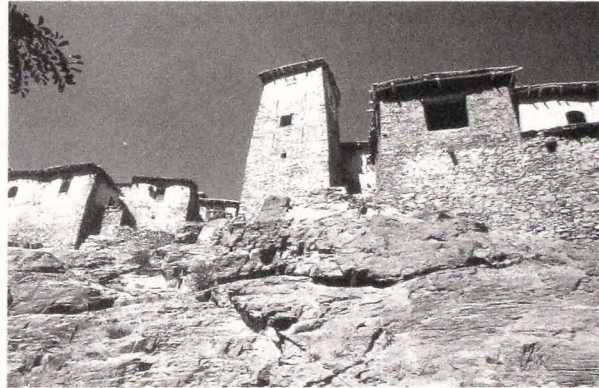
37. Village of flat-roof construction with massive stone walls in the Salang Mountains near Taqma.
