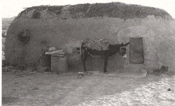
26. Completed kodik with a high threshold to deter snakes and illustrating the use of an unmudded roof to increase ventilation in the summer.
