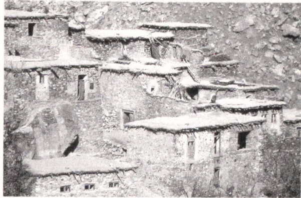
47. Detailed view of Taqma residential clusters with ladders for vertical circulation.
